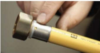
**4. ENSURE PIPE CAN BE SEEN THROUGH INSPECTION HOLE**
