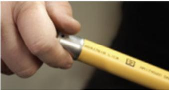
**3. FIRMLY PUSH PIPE INTO FITTING**
